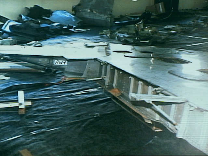
Structures 7 - RW-4 Photo 7
