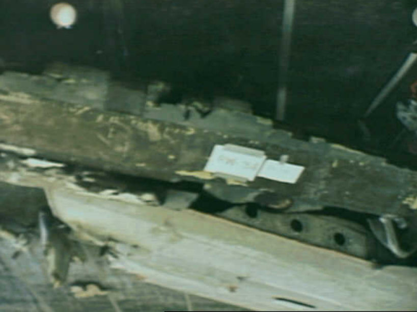
Structures 7 - RW-34 Photo 1
