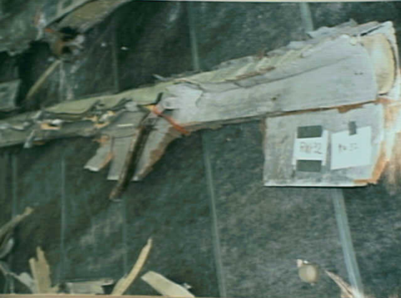
Structures 7 - RW-32 Photo 2
