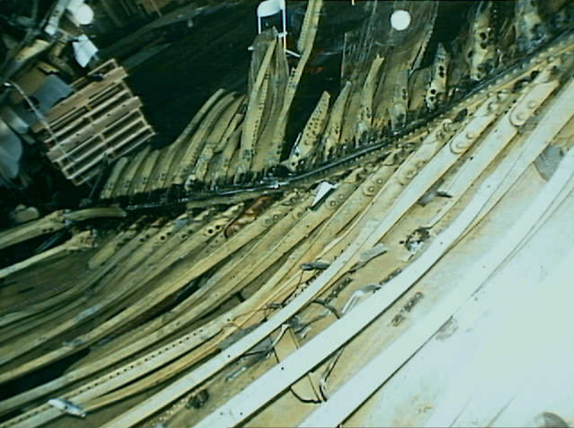
Structures 7 - RW-3 Photo 3
