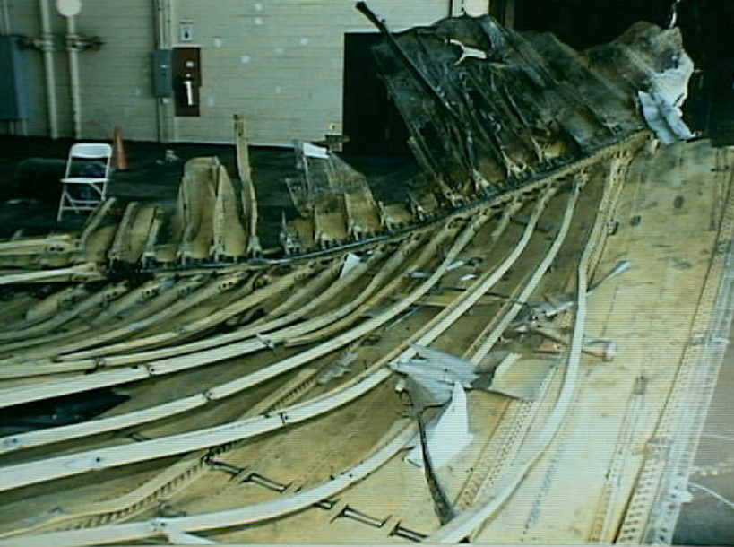
Structures 7 - RW-3 Photo 2
