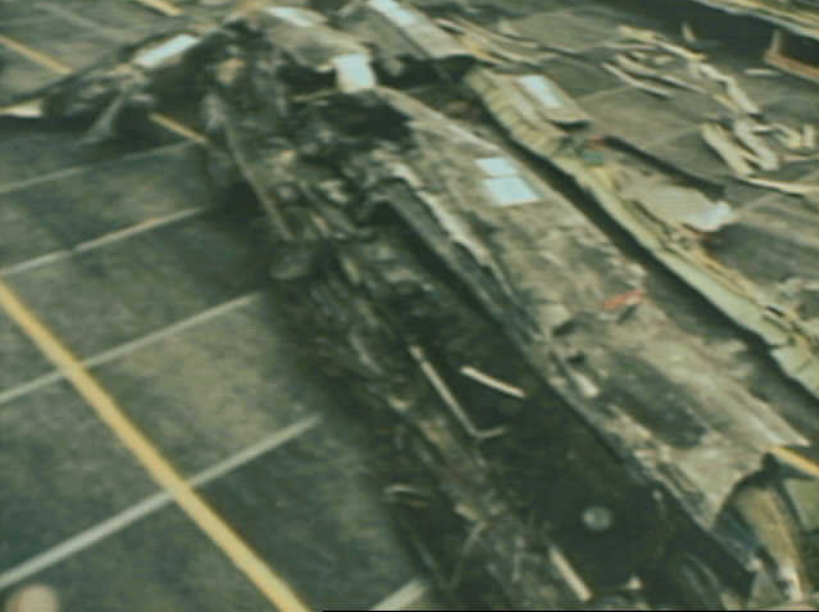
Structures 7 - RW-26 Photo 3
