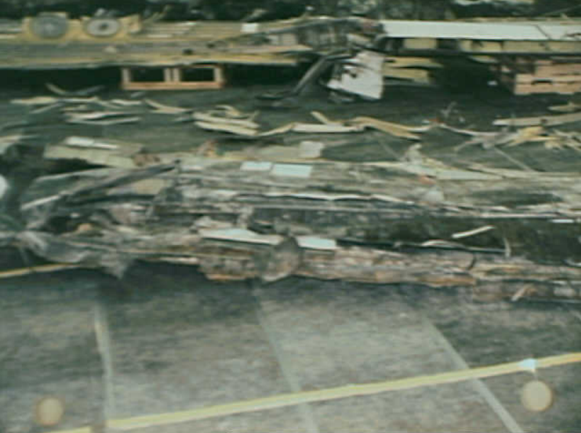
Structures 7 - RW-26 Photo 2
