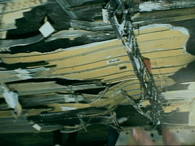
Structures 7 - RW-20 Photo 2
