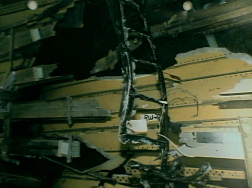
Structures 7 - RW-20 Photo 1
