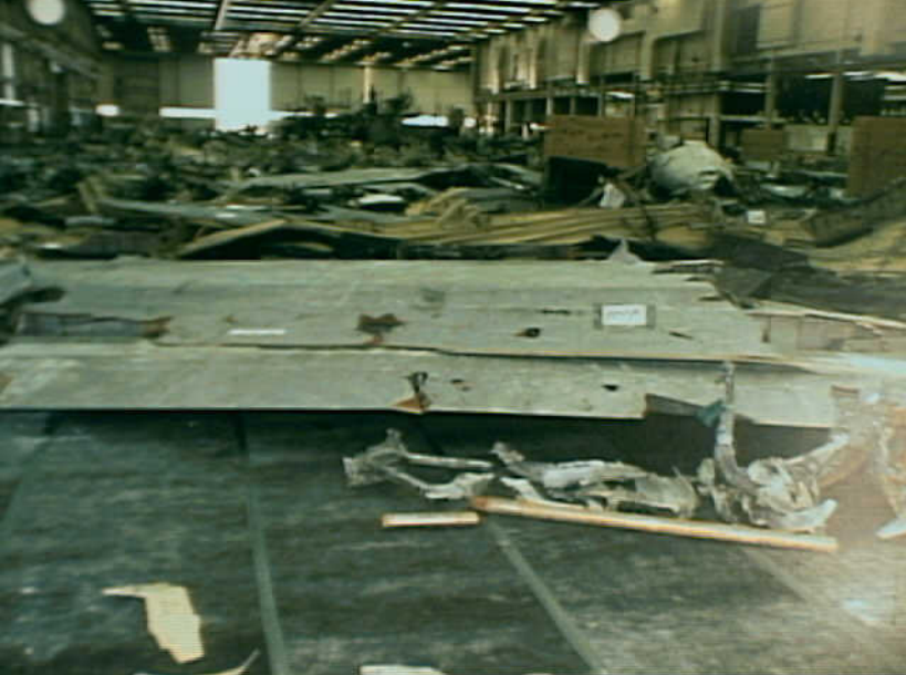
Structures 7 - RW-16 Photo 2
