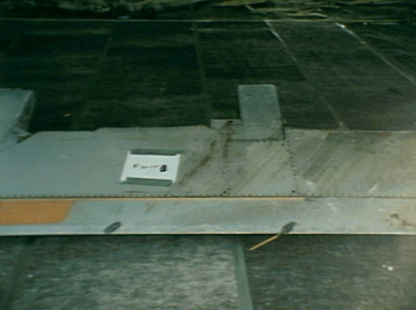
Structures 7 - RW-15 Photo 3
