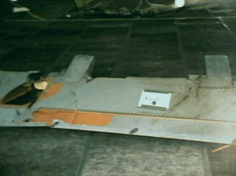
Structures 7 - RW-15 Photo 2
