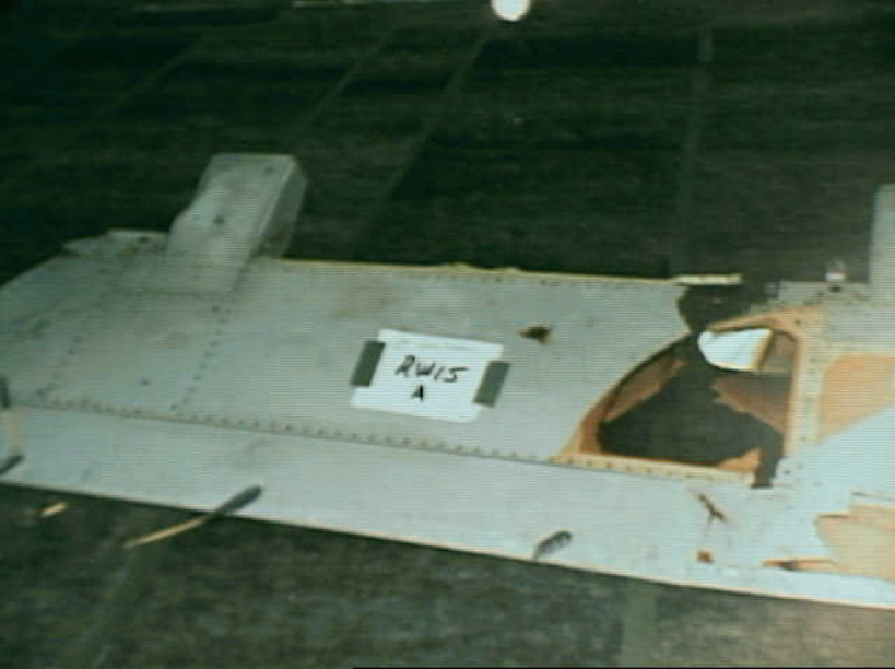
Structures 7 - RW-15 Photo 1
