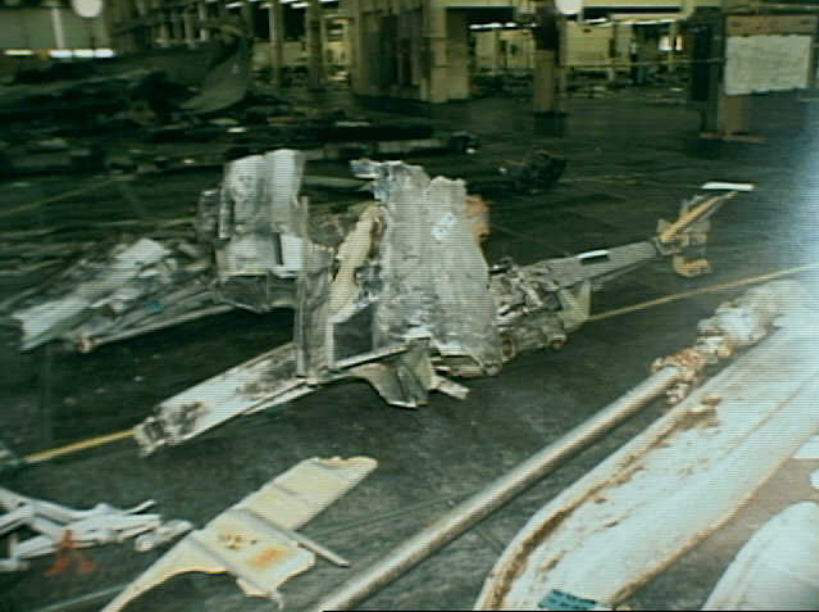
Structures 7 - RW-14 Photo 2
