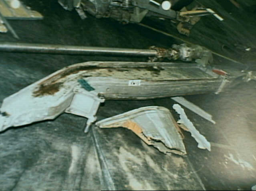
Structures 7 - RW-13 Photo 1
