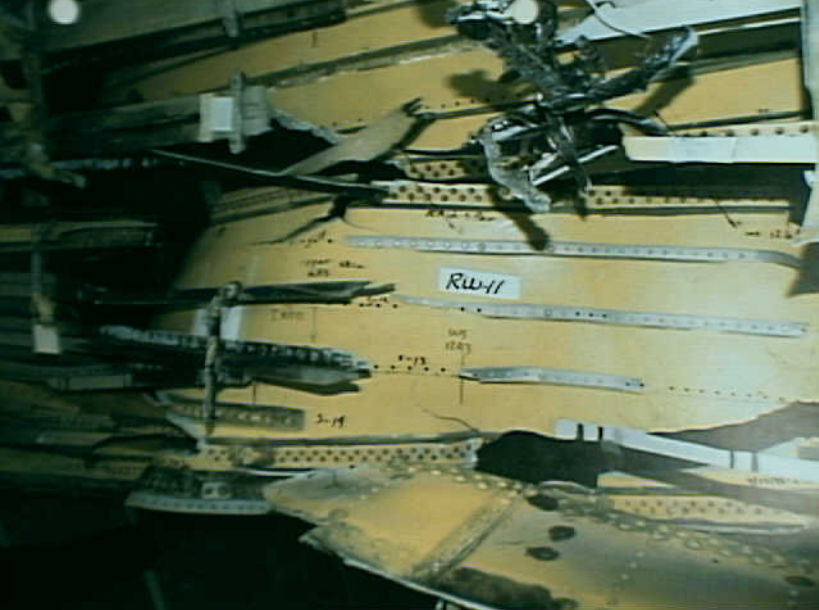
Structures 7 - RW-11 Photo 1
