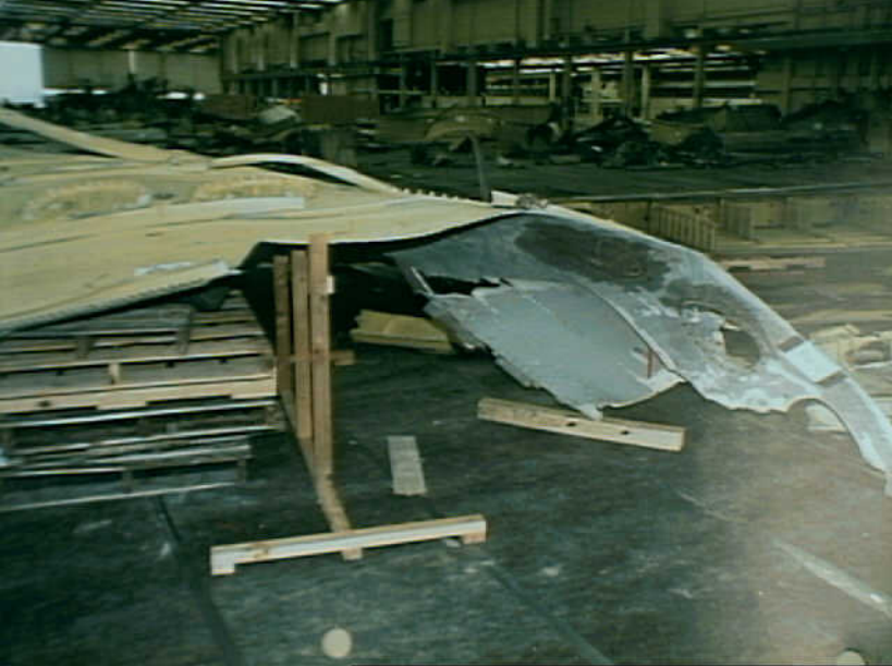
Structures 7 - RW-10 Photo 3
