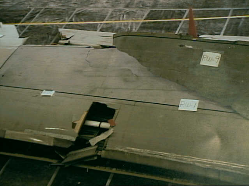
Structures 7 - RW-1 Photo 2
