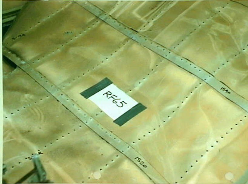
Structures 7 - RF-65 Photo 1
