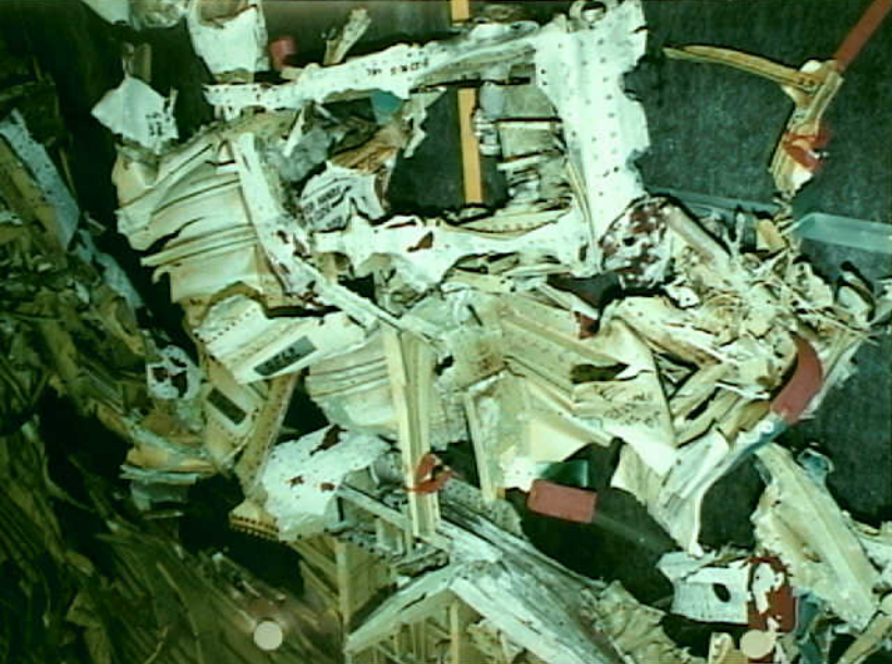
Structures 7 - RF-62 Photo 2
