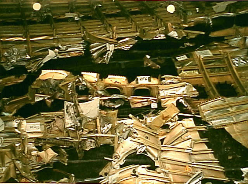
Structures 7 - RF-6 Photo 3
