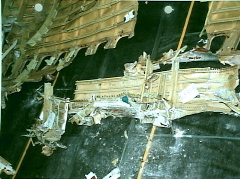
Structures 7 - RF-30 Photo 3
