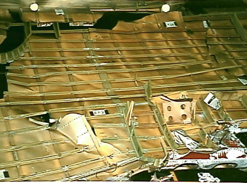
Structures 7 - RF-2 Photo 2
