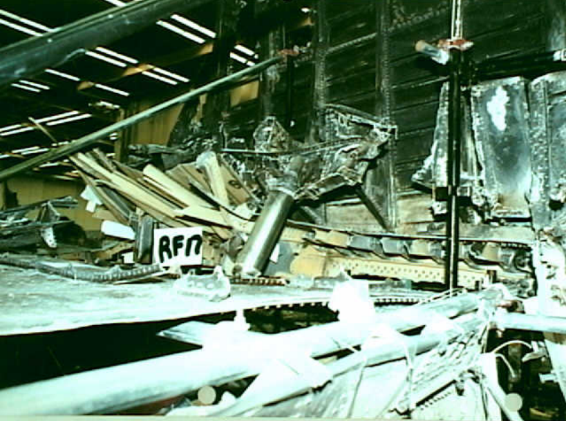
Structures 7 - RF-17 Photo 2
