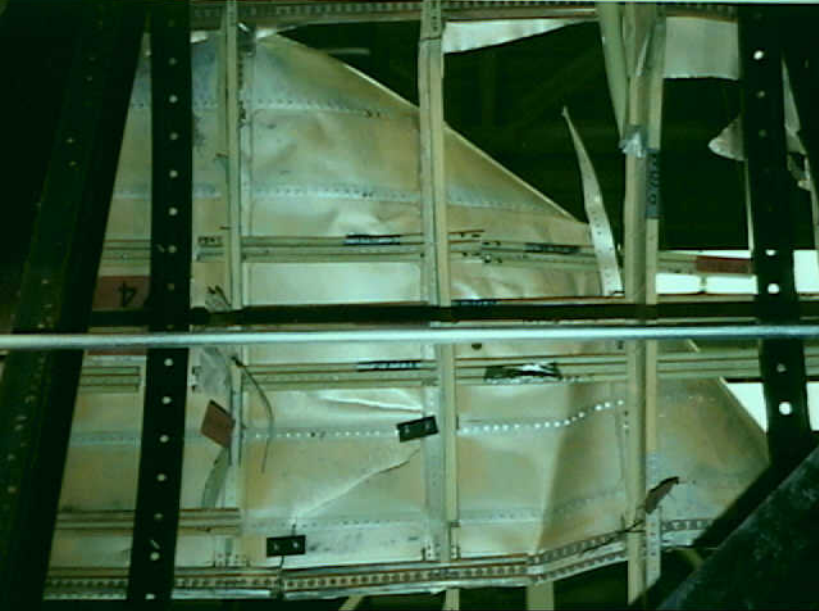
Structures 7 - RF-123 Photo 4
