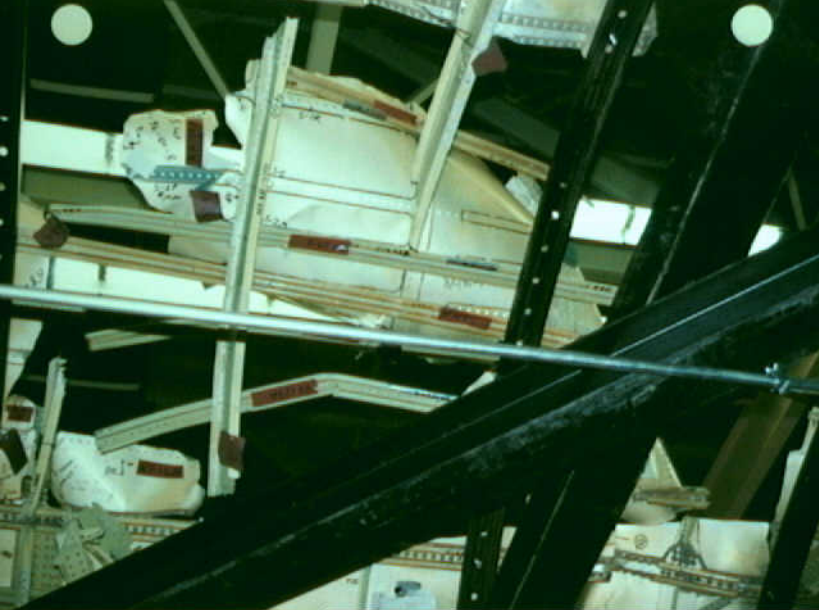
Structures 7 - RF-123 Photo 3
