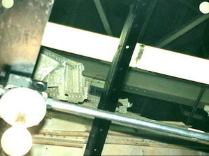
Structures 7 - RF-122 Photo 8
