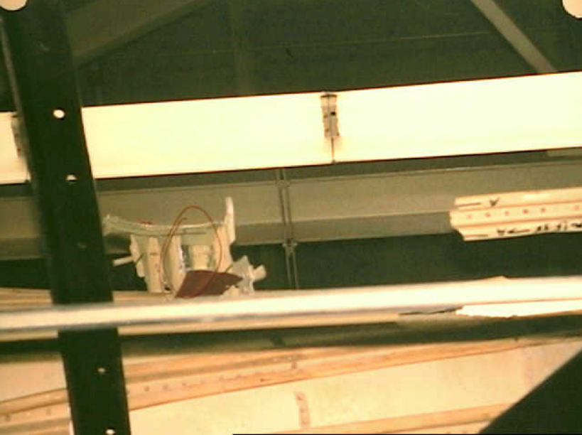
Structures 7 - RF-122 Photo 2
