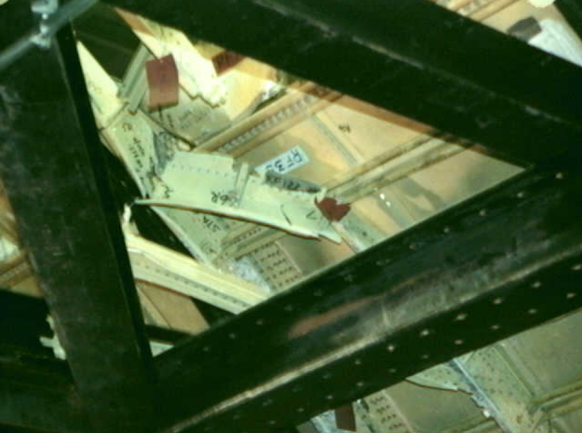
Structures 7 - RF-122 Photo 18
