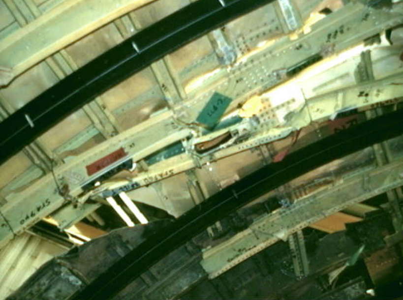
Structures 7 - RF-122 Photo 16
