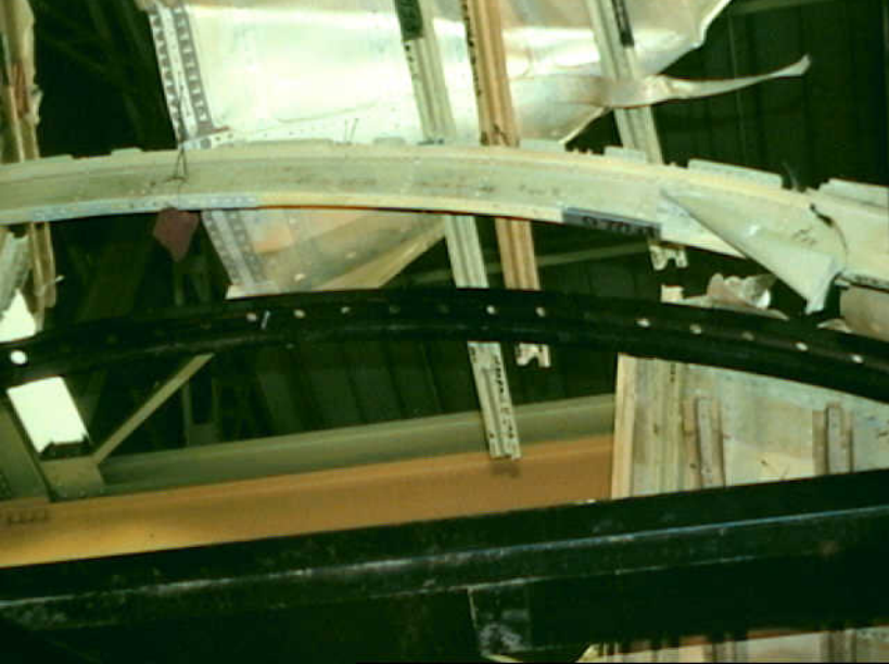
Structures 7 - RF-122 Photo 13
