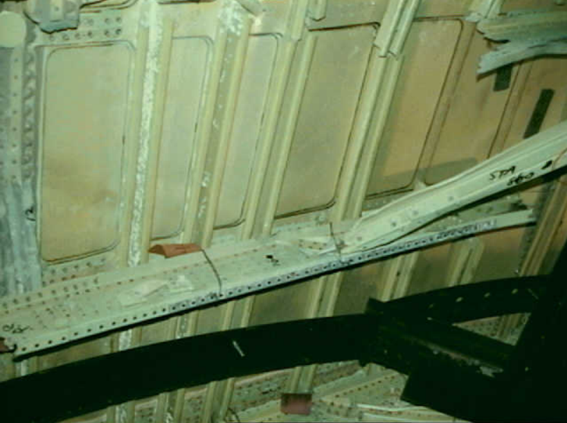
Structures 7 - RF-122 Photo 12
