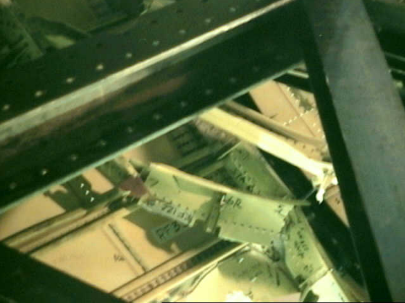
Structures 7 - RF-122 Photo 11
