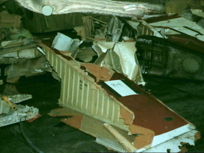
Structures 7 - R-4 Photo 2
