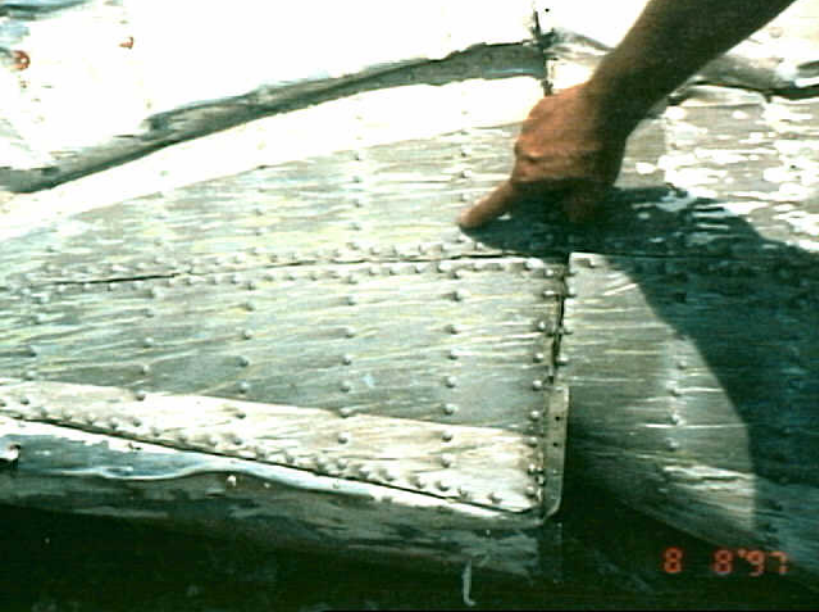
Structures 7 - Photo 8. View of the tail cone.
