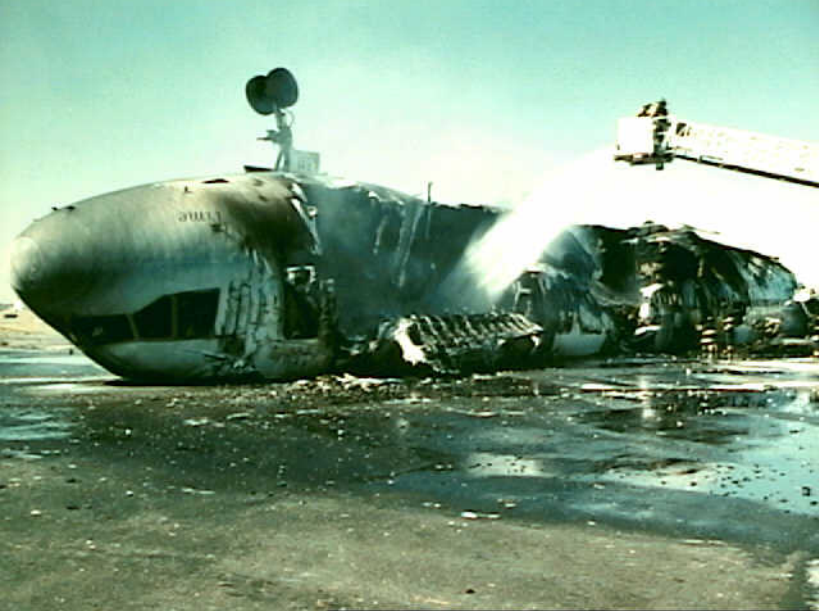
Structures 7 - Photo 2. View of the right side of the burned fuselage
