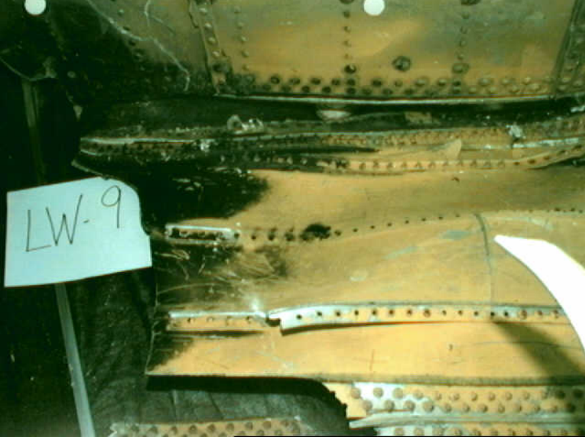
Structures 7 - LW-9 Photo 2
