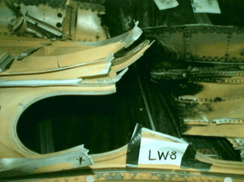
Structures 7 - LW-8 Photo 4
