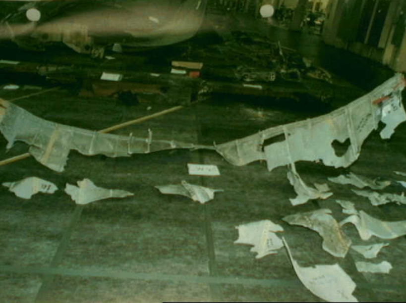
Structures 7 - LW-45 Photo 2
