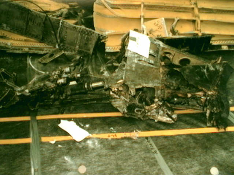
Structures 7 - LW-36 Photo 1
