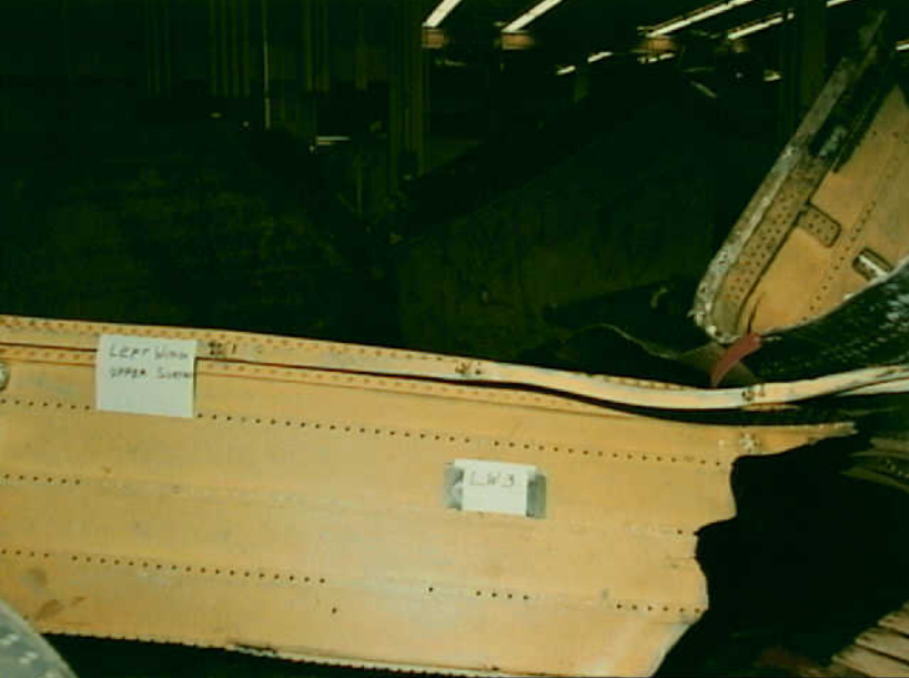
Structures 7 - LW-3 Photo 4
