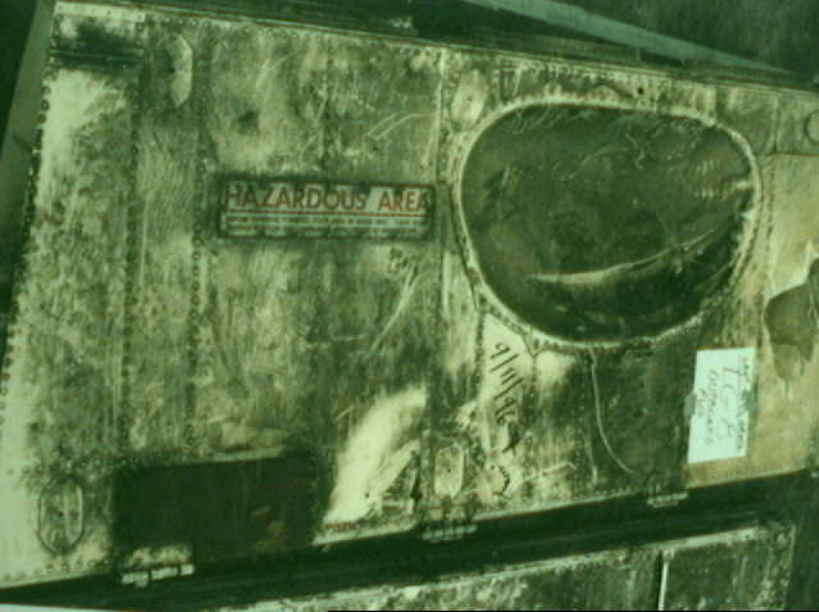
Structures 7 - LG-8 Photo 3
