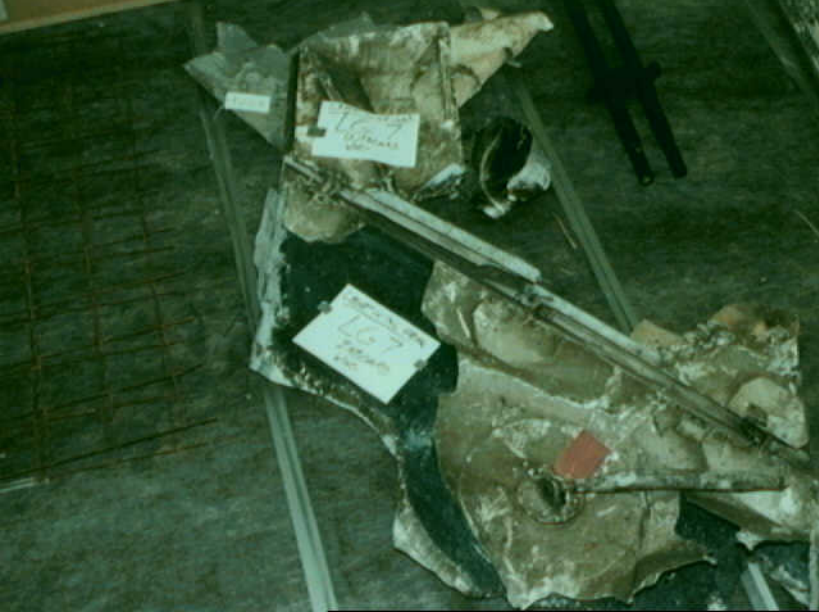
Structures 7 - LG-7 Photo 4
