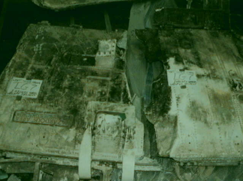
Structures 7 - LG-7 Photo 1
