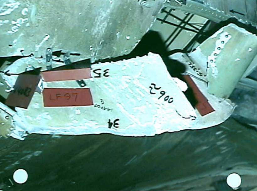
Structures 7 - LF97 - Photo 1
