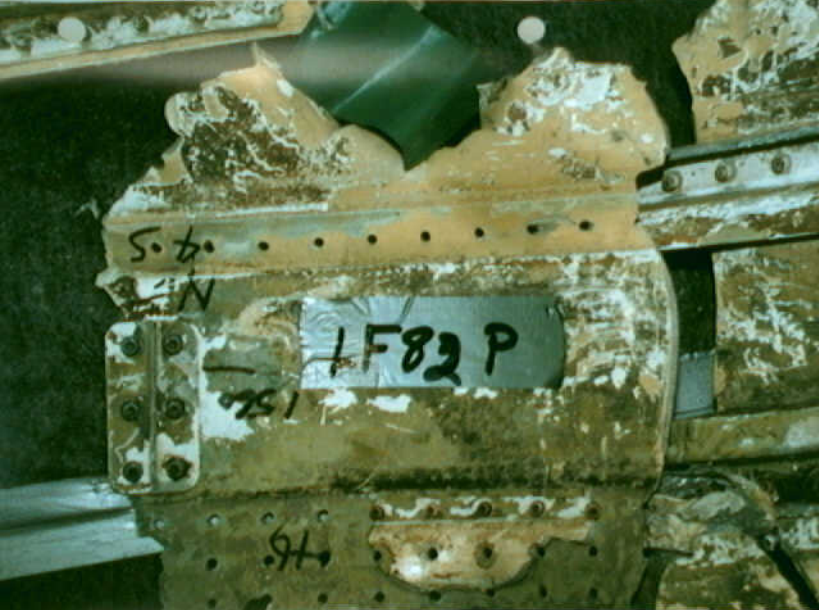
Structures 7 - LF82 - Photo 16
