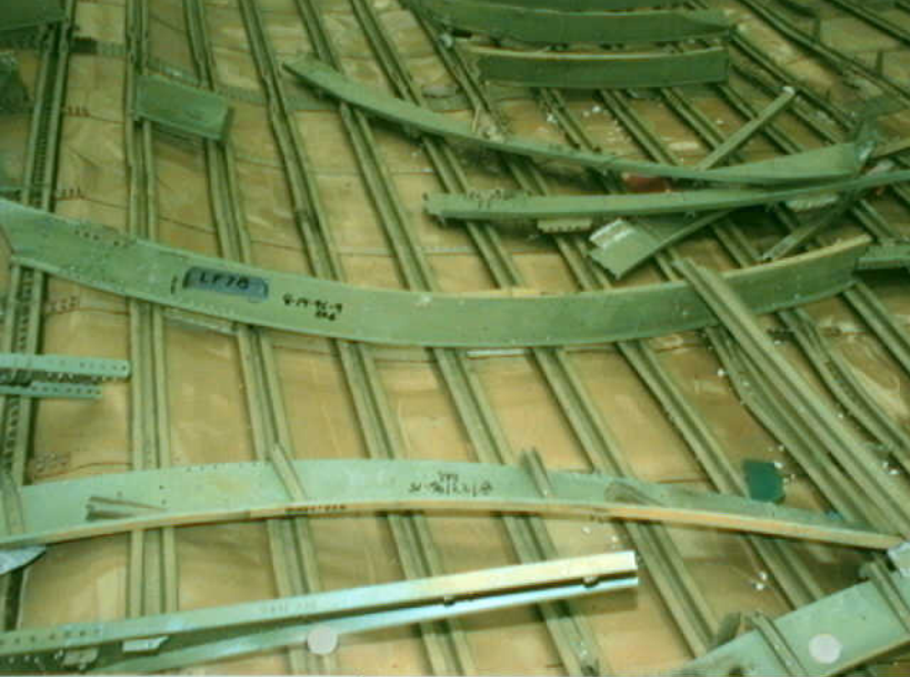
Structures 7 - LF78 - Photo 1
