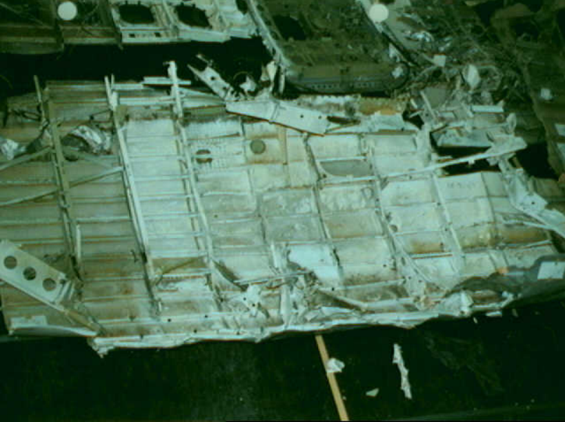
Structures 7 - LF7 - Photo 3
