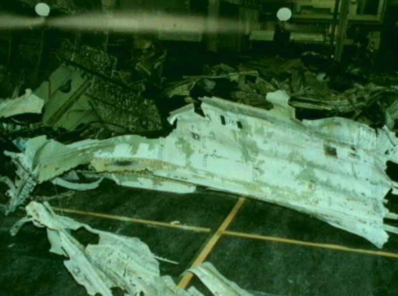
Structures 7 - LF41 - Photo 3
