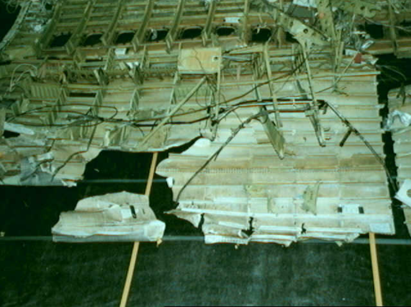
Structures 7 - LF4 - Photo 2
